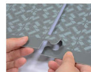
Step 6. Snap the structure in place
